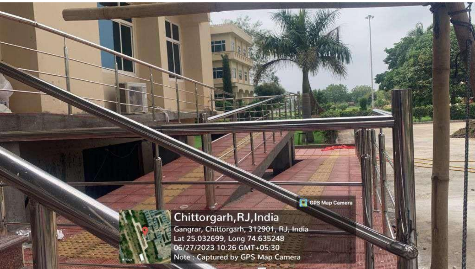
Ramp with railing for Easy Access
